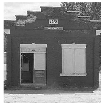
BELOW: Pre-restoration photos.
